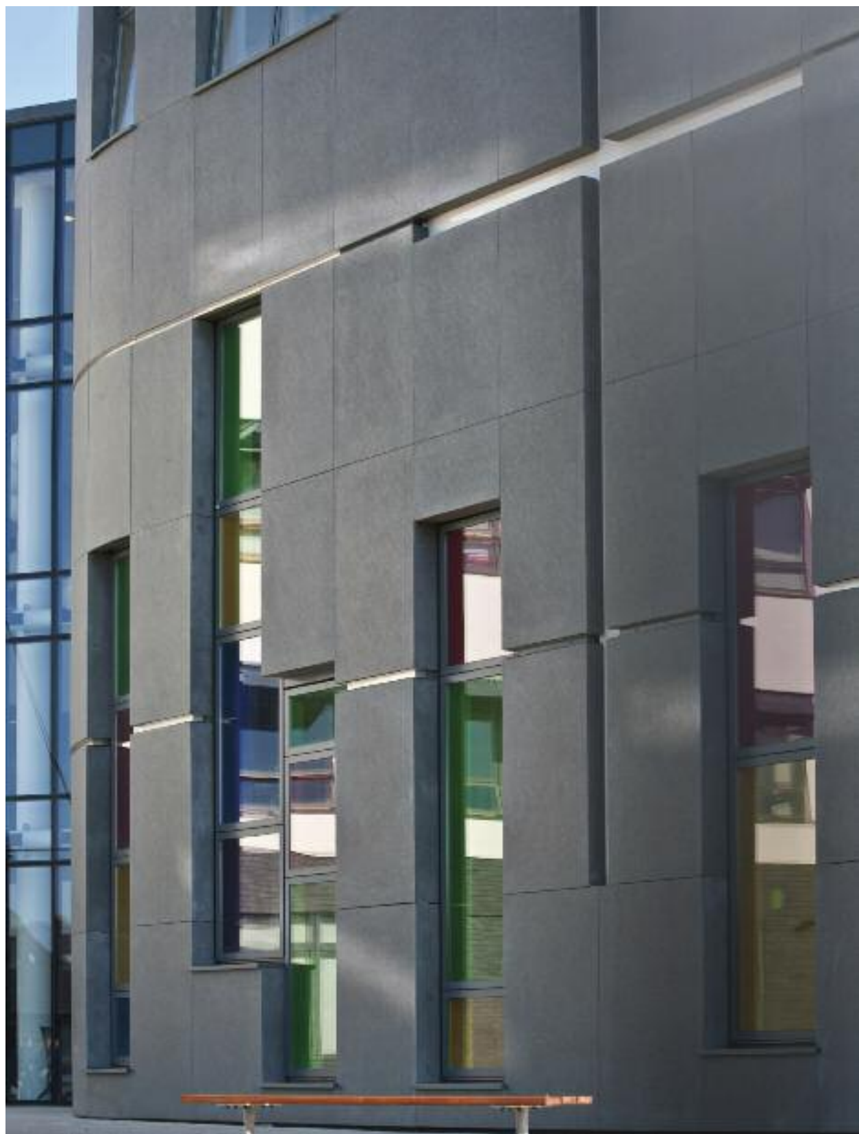
Ysgol Uwchradd Gatholig Archesgob McGrath, Pen-y-bont ar Ogwr / Archbishop McGrath Catholic High School, Bridgend
